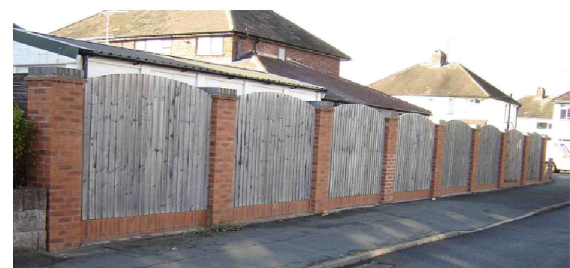
WALL WITH FENCE ABOVE
